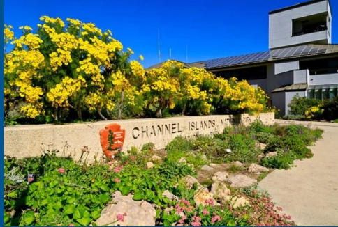
Channel Islands National Park Visitor Center Ventura Harbor
